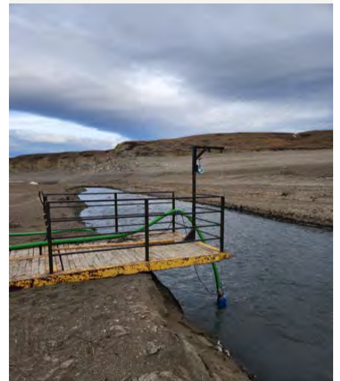
Emergency intake facility at the Oldman River Reservoir for nearby urban communities.
